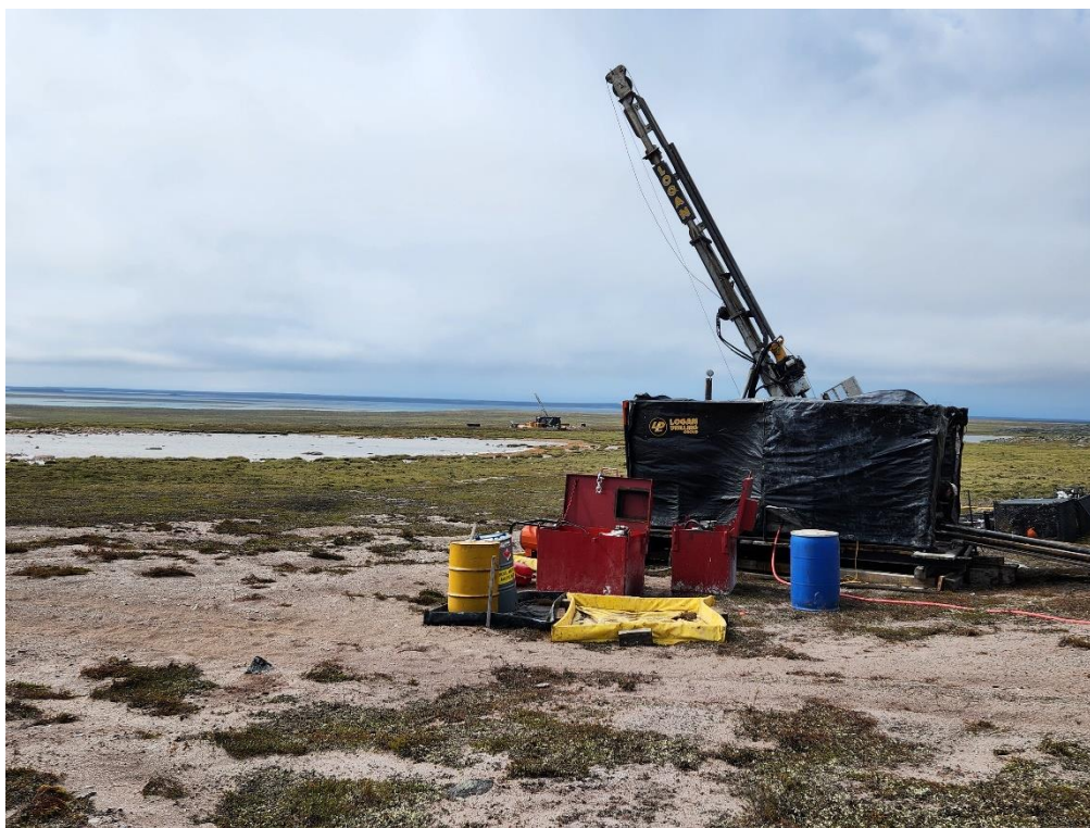
The second drill rig operating with the first drill in the background.
